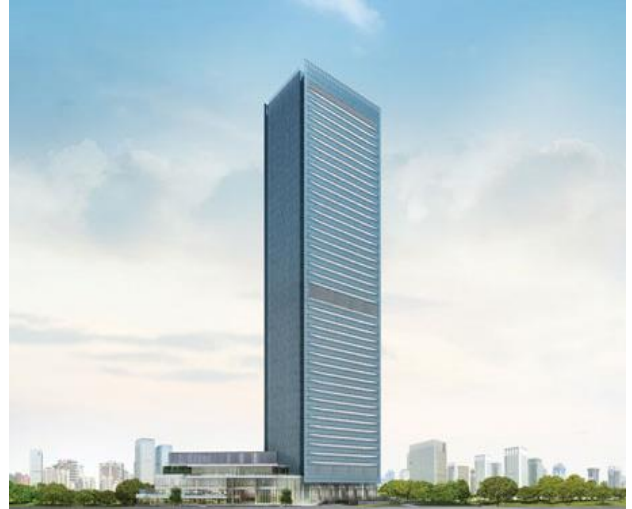
World Trade Center 3 Project – Jakarta
