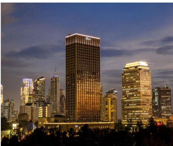
Fairmont Hotel Senayan Project- Jakarta
