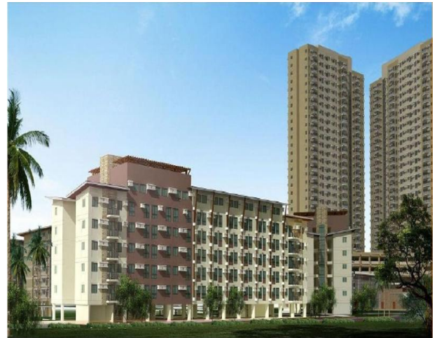
The Breeze Tower Project – Tangerang
